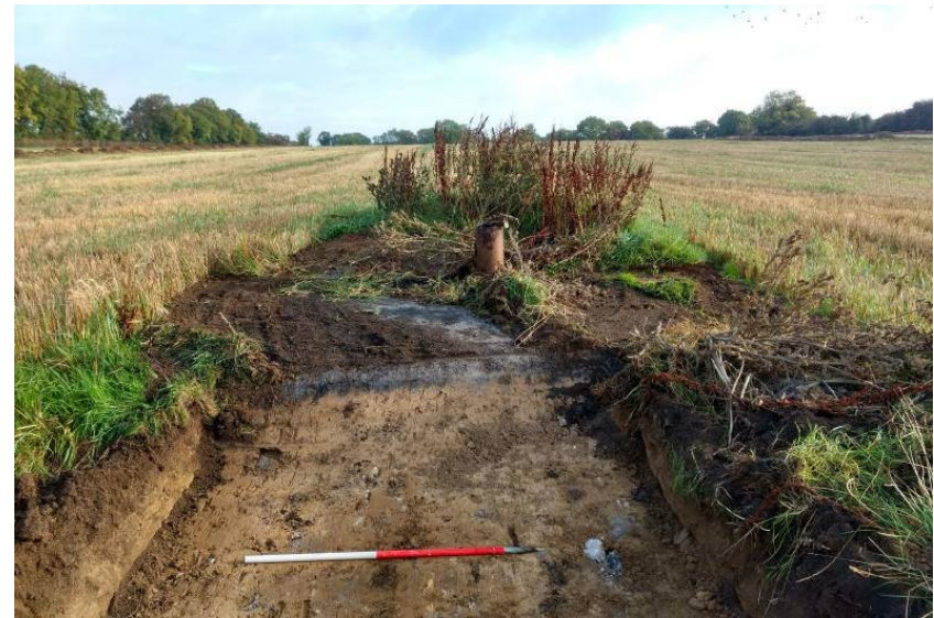
Plate 16 T21, manhole disturbance, facing northeast
