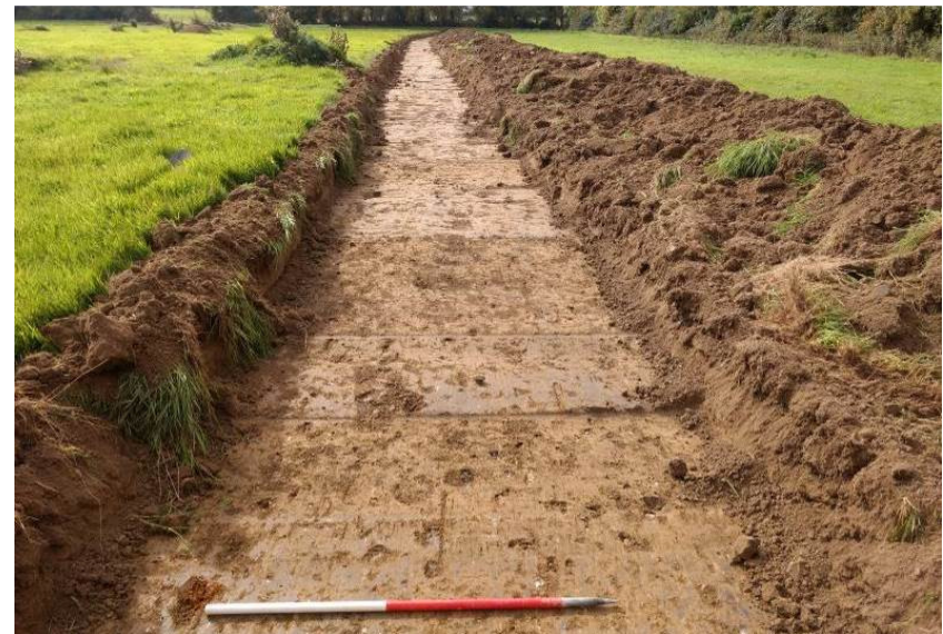
Plate 20 T30, facing southwest
